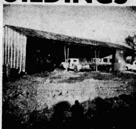
SHOP — 24x80x12-Ft. Located at the Wendell Moore Ranch, Merrill, Oregon. $2390.00 complete for all materials. Above building erected by owner.
