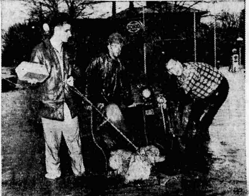
GRIMLY FAMILIAR are these scenes along the Ohio River and its tributaries, which often boil beyond flood stage in mid-winter. Damage in the Central States area from western New York to Indiana was estimated at more than 100 million dollars.
