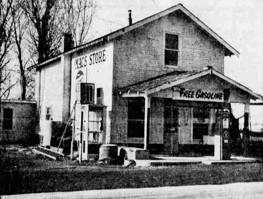
A LANDMARK in the Henley District is bowing to progress and is being torn down. This building was put up in 1912 by J. S. McClellan and was a meeting place for many years for neighbors. Mr. and Mrs. McClellan and their two sons, Verne, and Hugh lived in an apartment in the rear. Three sleeping rooms upstairs were rented to teachers who boarded with the family. The land on which the store was built was leased from John Koontz who homesteaded 88 acres about 1890. High school students in the Henley District then went to school until Christmas in Merrill, finished the rest of the year at the old Klamath County High School in Klamath Falls. Grade school students went to the Mt. Laki School, now the Henley Grange Hall.
