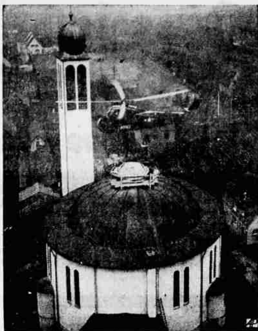
ARMY HELPS CHURCH — U. S. Army helicopter hoists 1,400-pound plastic cupola atop roof of circular-shaped Catholic church at Mussbach, West Germany.
