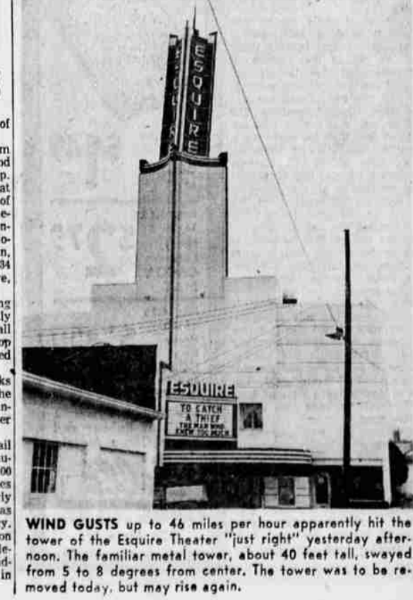
WIND GUSTS up to 46 miles per hour apparently hit the tower of the Esquire Theater "just right" yesterday afternoon. The familiar metal tower, about 40 feet tall, swayed from 5 to 8 degrees from center. The tower was to be removed today, but may rise again.
