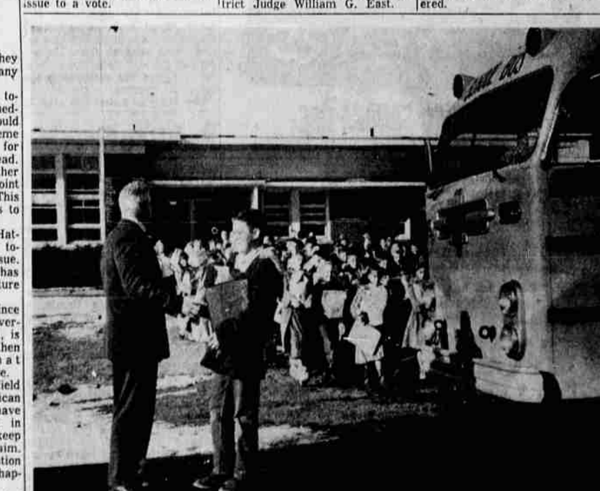
HEADING for the new Orson A. Stearns School at Laverne and Crest were these students from Peterson School. Students numbering 150 were transferred by bus to the new school. Here, in foreground, Peterson Principal Art Millard directs the loading process. Pupil Danny Nelson is all set for the move, loaded down with books and supplies.
