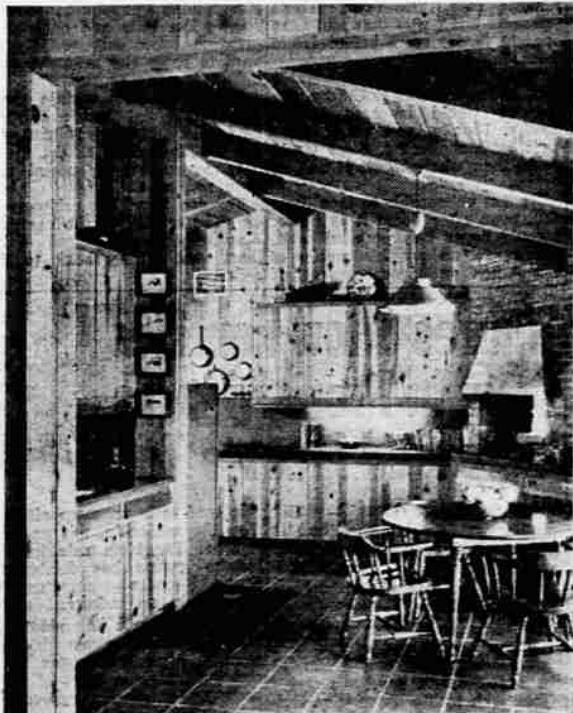
PANELING FOR FAMILY ROOM — Knotty paneling from the Western pine region provides the attractive warmth and interest to this family room which connects kitchen, bar, dining, and barbecue areas. The walls are six-inch wide inland red cedar and the ceiling random width cedar with Douglas fir beams. The wood is all finished with natural lacquer and wax.
