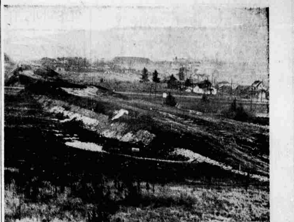
WORK IS MOVING SWIFTLY on the grading portion of the west side bypass. This picture, taken from U.S. 97 north of Kit Carson Way and looking south toward the gap at Oregon Avenue, clearly shows the progress on this bypass route. If the weather continues favorable for construction, grading on the bypass may be completed in January next year. L. Rogers Construction Company of Portland has the grading contract. Contracts have also been let for all the structures of the bypass. The gap can be seen where a bridge will span the Southern Pacific tracks. — Photo by Otto Ellis
