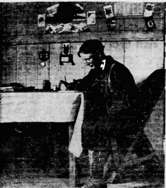
THE STATION AT POKEGAMA was headquarters for a two man fire fighting crew in the early days of KFPA. Here Hal Ogle, present district warden, is pictured at one of the rude tables filling out his daily report. He was stationed at Pokegama with Roy Hackard, now dead, both under the supervision of Jack Kimball. — Photo from Ogle
