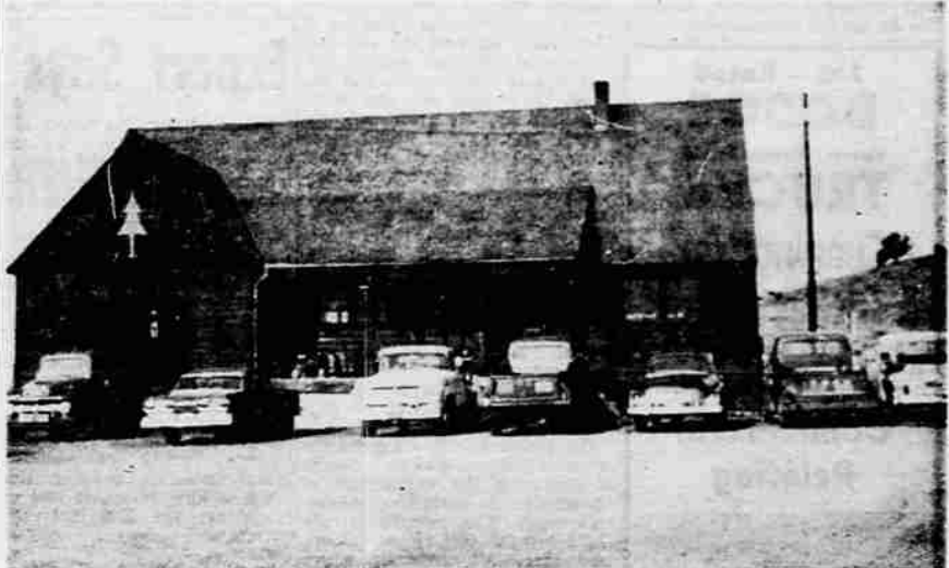
THE SUPPLY SHED at KFPA offers a wide assortment of fire fighting tools when an emergency arises. The building is shown here with a few of the outfit's trucks standing ready in case of call. The headquarters are located at the Weed-Ashland junction.
