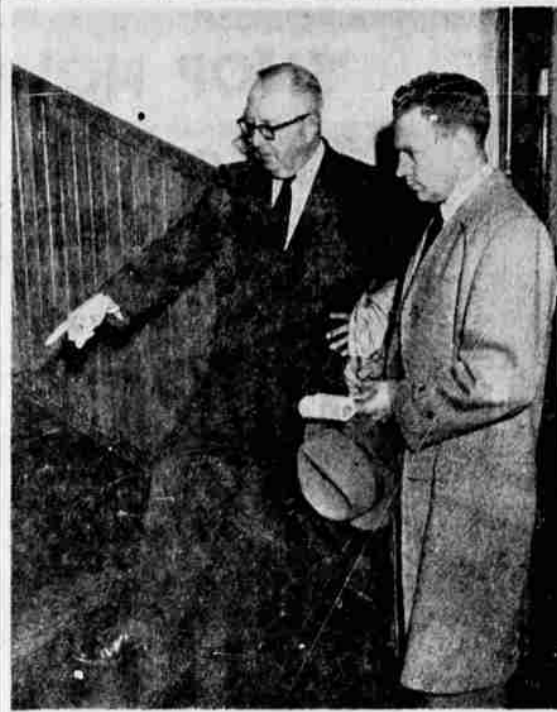
RIVERSIDE SCHOOL was inspected Tuesday afternoon by Deputy State Fire Marshal Wilburn R. Dodge who is looking at one of the staircases being pointed out by School Superintendent Arnold L. Gralapp. Some of Dodge's first reactions to the school, which has been described as containing fire hazards by City Fire Chief Roy Rowe are given in the story on Page 4.
