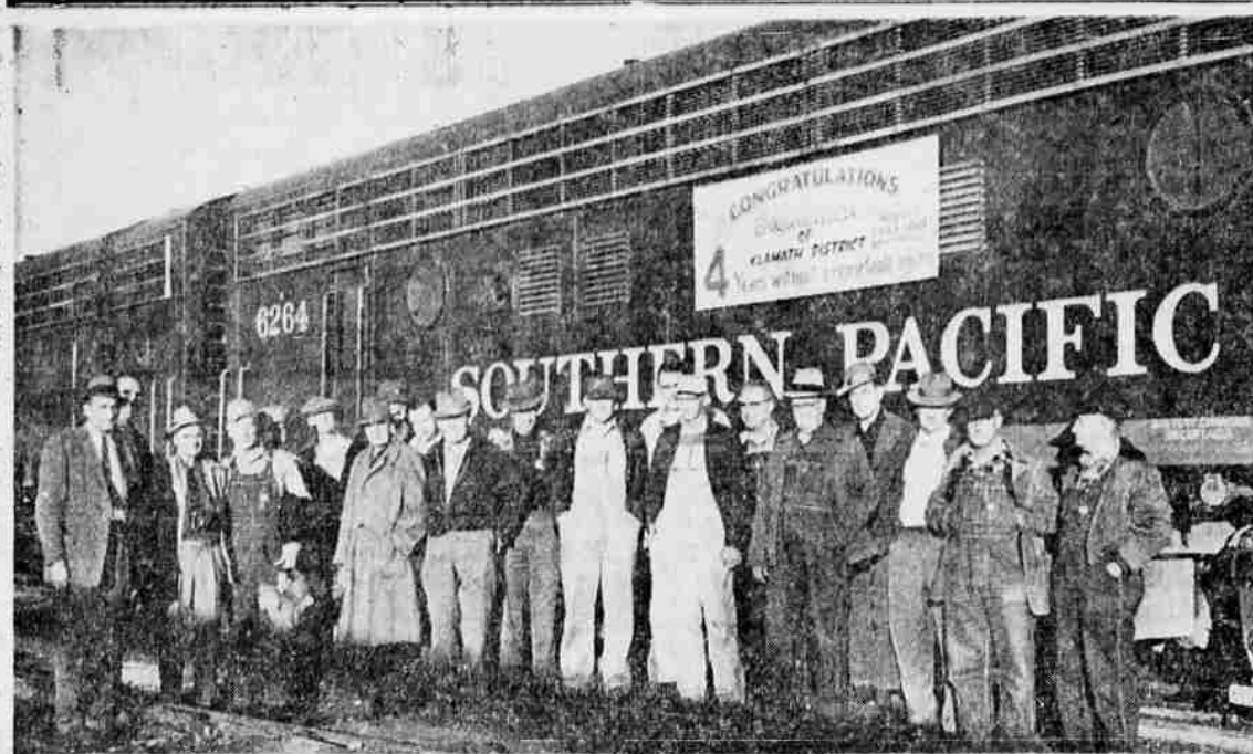
UNEQUALLED SAFETY RECORD in the history of the Southern Pacific Company has been made by this group, according to announcement by R. R. Robinson, superintendent of the SP Shasta Division. These men completed four years of service on November 26 without a single personal injury in connection with their employment. Robinson stated: "It proves a job know-how and performance in the highest tradition of good railroading." Shown from left are R. M. Dickson, road foreman of engines in charge of
