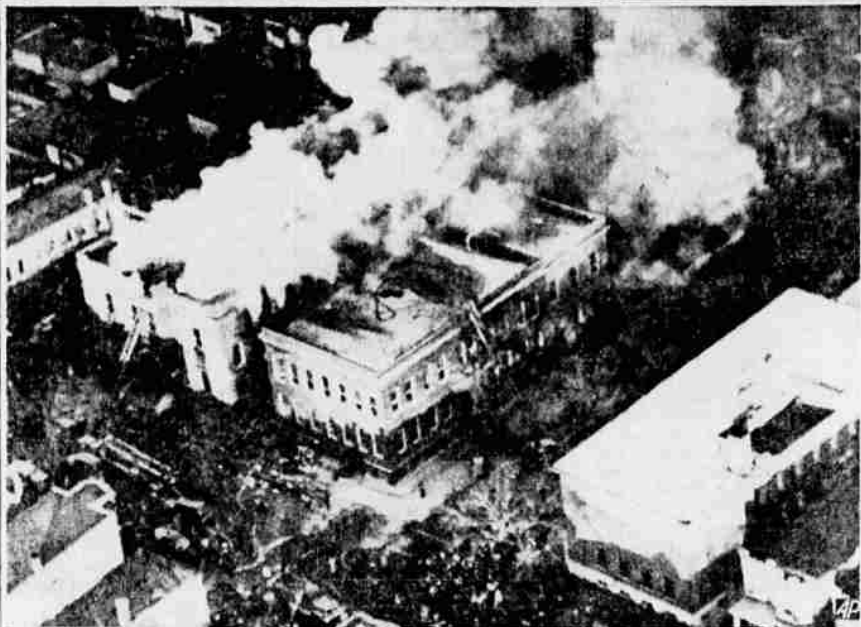
FLAMES ENGULF CHICAGO SCHOOL, Our Lady of Angels parochial school, in the fire that claimed more than 80 youngsters and three nuns. Most of the casualties were on the second floor.
