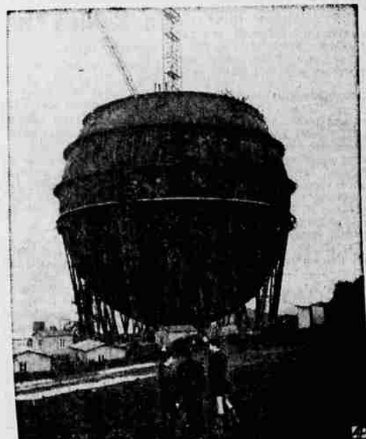
RUHR SIGHT — Youngsters eye giant spherical gas storage tank under construction at Wuppertal, Germany. Steel tank will have capacity of 8,000,000 cubic feet.
