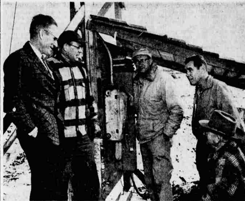
FIRST CUSTOMERS of the South Suburban Sanitary District were expected to be served today by the vast sewer facility nearing completion. Installation of electric pumps was completed when this group of men pulled the switch and found things in perfect working order. Left to right are Carl Yancey, district director; Fred Lewis, president of the board of directors; Morris D. Gunderson, project engineer; Harold North, office manager, and Walter Nitzel, director.
