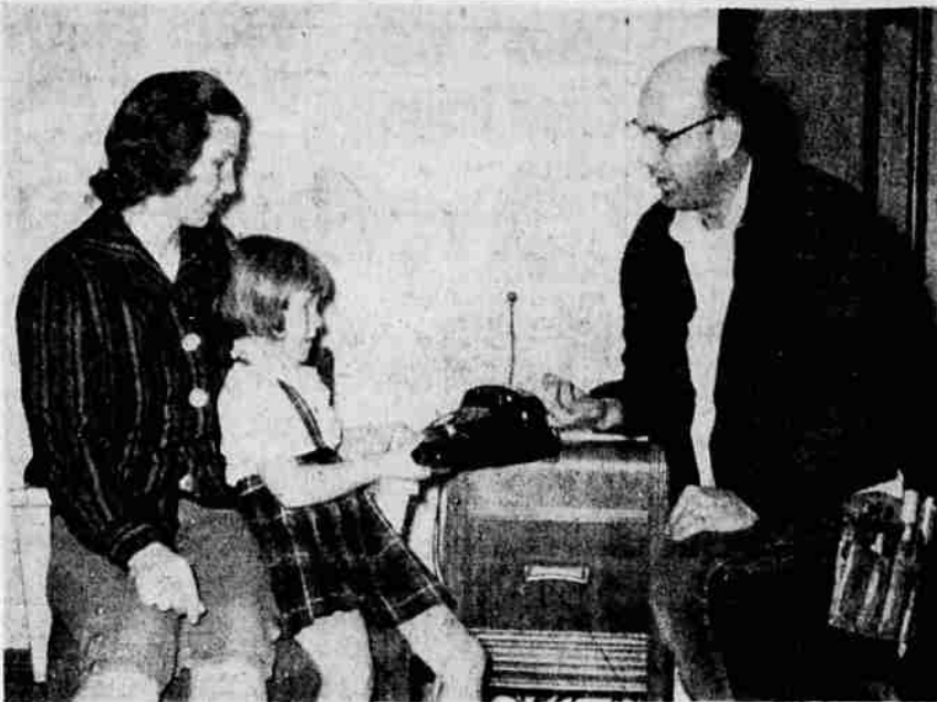
THE FIRST TELEPHONE was installed in the new Kingsley Field housing facilities on Monday, November 10. Here, Harold Rush, installer, is busy hooking up a new color set and a bedroom extension in the home of S. Sgt. and Mrs. Jack F. Lair, 822A Kincheloe Avenue. Sergeant Lair is a career man in the armed services, having 12 years in the medical supply section of the Air Force. Mrs. Lair is a former telephone operator for the General Telephone Company of the Northwest at Bonners Ferry, Idaho.
