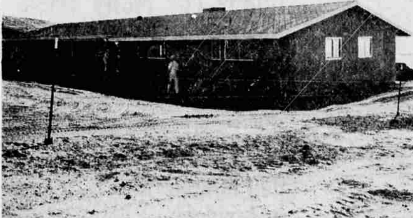
WORKMEN PUT OUTSIDE TOUCHES on this four bedroom, single unit which will be occupied by the base commander, Colonel Jack Williams. It is expected to be ready for occupancy shortly after the first of the year. The commander's home is located at the corner of E street and North B Avenue.
