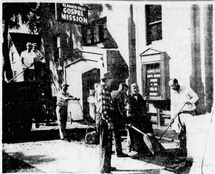
BLACKTOPPING MATERIAL , donated by the Clemens Construction Company of Klamath Falls and Tulelake, has been used to surface the sidewalk around the Klamath Falls Gospel Mission. The material was hauled to the Mission in a truck donated by the Bly Logging Company. Men in the picture not identified stopped by to offer assistance. On the ground, left to right, are Jack Wright, with the roller, assistant superintendent at the mission, John Pederson, superintendent; Clarence Stengle, staff member at the mission, unidentified man, and Mac Bryan, truck driver for Morrison Knudsen Construction Company.
