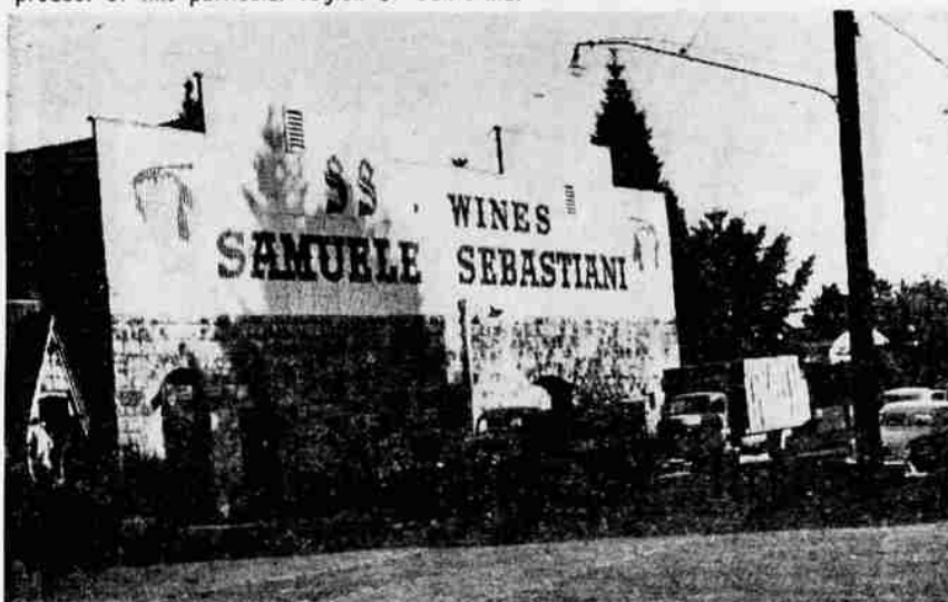
SAMUELE SEBASTIANI produces some of the best wines you will ever find and boasts an outstanding panel of winners over the years. This picture shows the front of the winery building, the retail room at the left and the offices at the right behind the trucks. At the extreme left is the shrine pictured on the cover. The winery is located just on the edge of Sonoma.
