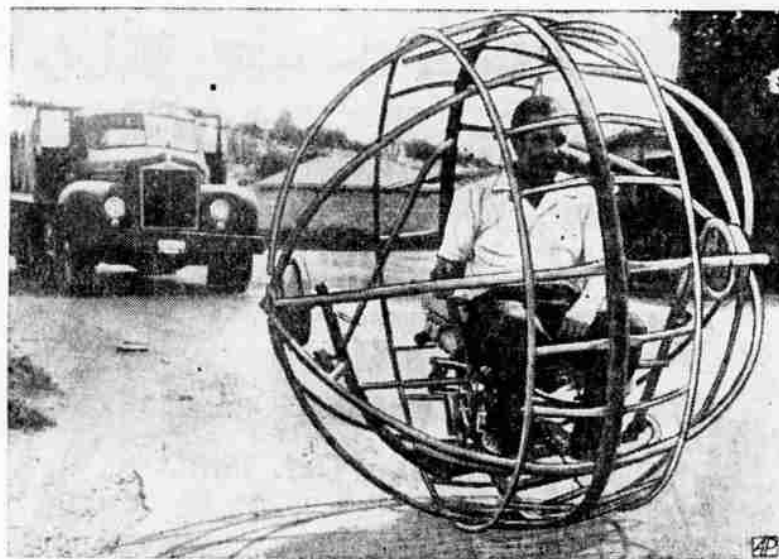
THINGS TO COME? — Herman F. Anderson demonstrates experimental model of his "car of the space age" in Nashville, Tenn. He says static tests show such a machine is capable of 200 miles an hour. Model is powered by a three horsepower lawnmower motor.
