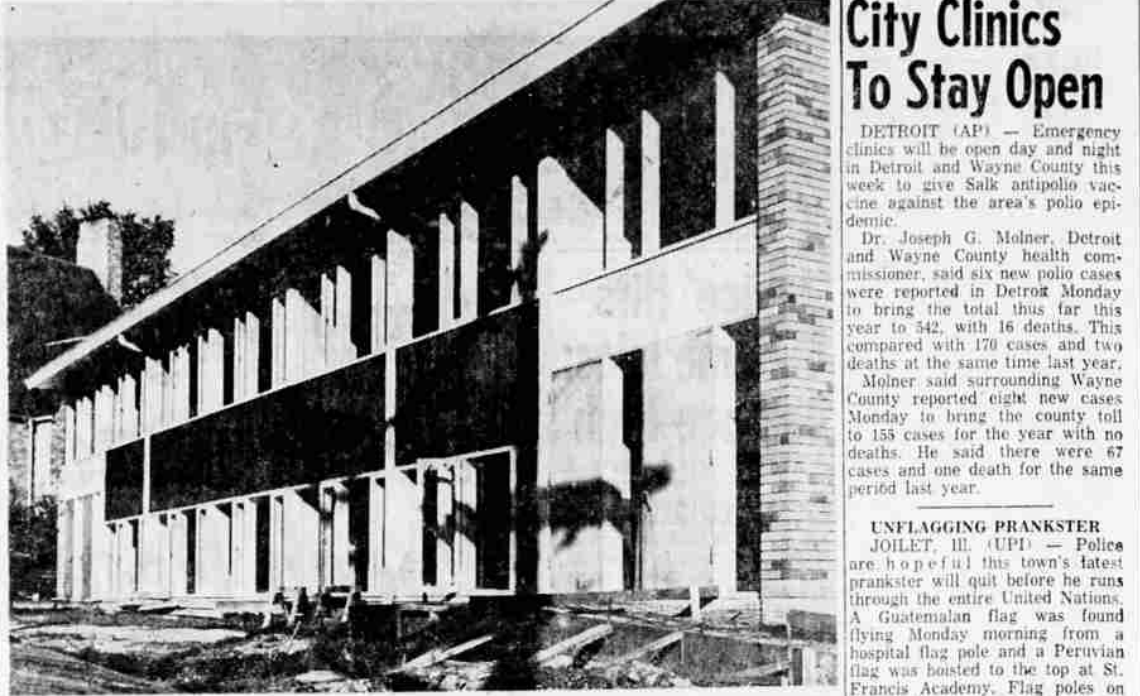
THIS NEW WING of the Klamath Lutheran Church was dedicated during the morning service Sunday, October 5, by Dr. H. L. Foss, Seattle, pastor of the Evangelical Lutheran Church, that city. The choir sang two appropriate numbers under direction of Stephen Stone. The two-story, brick and frame structure, with 6,300 square feet of floor space provides for 21 Sunday school rooms, two large assembly rooms, rest rooms and kitchenette on the second floor. Morrison and Howard were the architects. Eldon Alt was the contractor. Approximate cost of the structure including a covered walkway to be built between the wing and the main building is $77,000. First Sunday school classes in the wing will be held at 9:30 a.m., Sunday, October 12. Worship services will be at 9:30 and 11 a.m.
