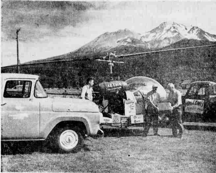
GROCERIES BY HELICOPTER are rushed to the crews completing the million dollar recreational facilities at the Mt. Shasta Ski Bowl. The 12 miles of all-weather highway being constructed by the U.S. Bureau of Roads to the bowl site is now in the last stages of completion and had to be closed temporarily. Rather than pull off crews painting and installing equipment in the $250,000 lodge, Carl McConnell, lodge contractor, resorted to air service to keep them supplied. From the left, the unidentified pilot of the helicopter; Bill diCristina, lodge manager, and McConnell.
