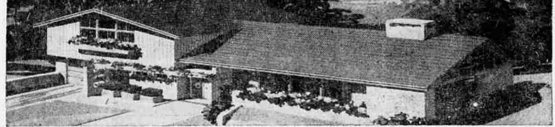
THIS RANCH-TYPE SPLIT will fit the personality of any owner because it has a large select-your-plan area adaptable to the special needs of any individual. The floor
