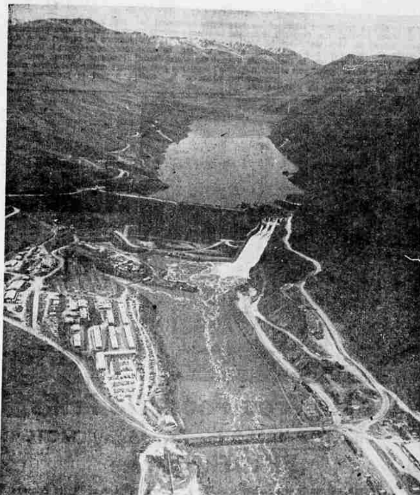
STOREHOUSE FOR WATER . . . Snake River water that will spin Brownlee Dam's turbines is seen in this aerial view filling the reservoir behind the huge rock-filled embankment, center, of Idaho Power Company's new 360,000 kilowatt hydro project. To the right of nearly completed embankment, spectacular concrete spillway is discharging water through three low level gate openings. The powerhouse, left center, is expected to be ready for production by September. Extending 57 1/2 miles upstream, the reservoir will have a storage capacity of 1,500,000 acre-feet of water, with one million acre feet usable each year for power, flood control and navigation.
