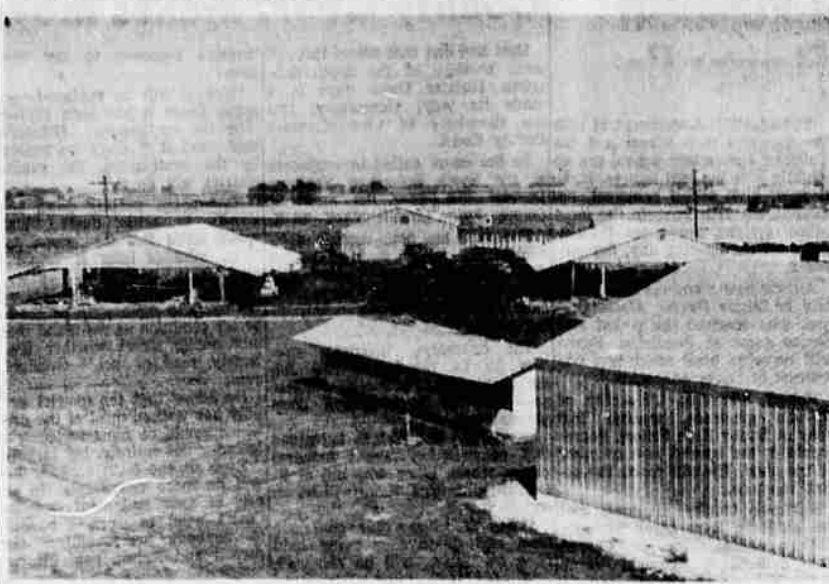
AREAS WITHIN the boundaries of the Tulelake-Butte Valley Fairgrounds at Tulelake, not under lawn and buildings, has been blacktopped by the Clements Construction Company of Fremont, California. In the foreground is part of the 35 acres of thick lawn, a feature that makes the fairgrounds one of the most attractive in California. Buildings are some of the livestock barns, a concession and exhibit building. Fair dates are from Friday night, September 5, through Monday, September 8, and the climax of the junior livestock show.
