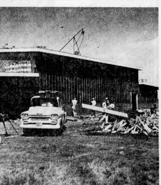
HENLEY SCHOOL ADDITION may be completed before the October deadline as work progresses on the $71,134 multipurpose unit to house a kitchen, cafeteria and some physical education facilities. Employees of Riverman and Sons, Portland contractors, are raising the brick veneer on the addition designed by Howard R. Perrin to conform with existing Henley School buildings. Construction began early in May.
