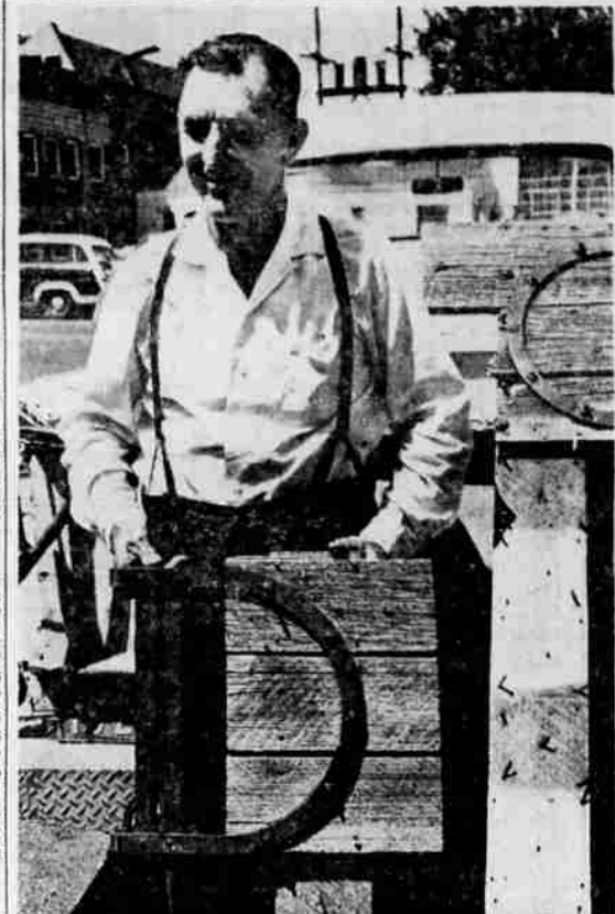
VACLAV KALINA , who has lived nearly half a century in Malin, displays part of a track once used in a horse barn on the Dalton Ranch near Malin, used to move hay to the animals tied at mangers. The metal was beaten out, probably by the ranch blacksmith. Nails dotting the timbers are handmade square nails. Timbers from the old barn and from other sources on the ranch will be used Sunday to cook beef for the Elks barbecue.
