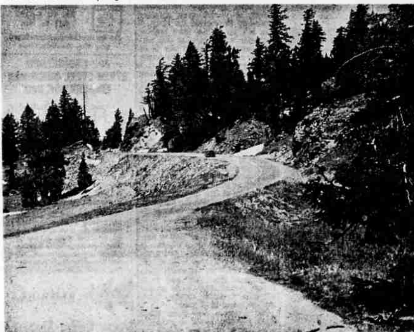
LONG, SWEEPING CURVES with timber creeping down to road's edge, snow lurking in the shadowed depths, make a cooling respite from summer heat for those who drive the loop road around the rim of Crater Lake during the summer and fall months. Many vistas open up to the driver to afford him glimpses of wild flowers, mountain meadows and long vistas to far-off mountains.
