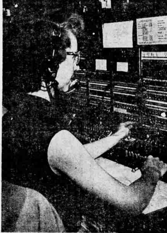
AT THE CENTRAL OFFICE of Pacific Telephone Company in downtown Klamath Falls Shirley Hill, mobile service operator, is shown about to plug into a special jack at her section of the switchboard to complete a mobile telephone call. From one to three operators, especially trained in mobile telephone work, are on duty at all times. There are in the neighborhood of 20 mobile telephone service customers registered in the Klamath Falls area. Each installation is assigned its own mobile telephone service number.
