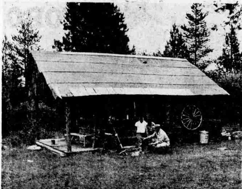
HEADQUARTERS FOR YMCA Camp Totton is this well-maintained, authentic old log cabin. Its maintenance is one of the projects of the "Y's Men," a group of young men affiliated to the "Y." YMCA Director Paul Campbell, right, who is in charge of the camp, explains some points of campcraft to, left to right, Jim Walker, Billy Cool and Carl Pepper.
