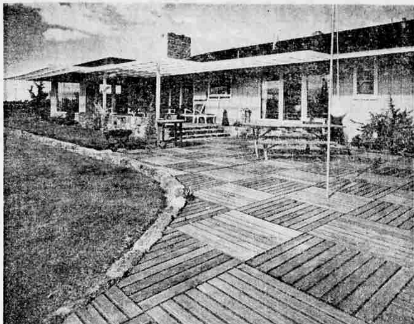
INTERESTING EFFECTS in patio design may be achieved with lumber from the western pine region. This attractive and practical patio for enjoyable outdoor living was constructed with squares formed by Douglas fir 2 by 4's nailed onto 1 by 4-inch cleats. The wood was treated with a pentachlorophenol preservative to provide resistance to decay. Note the use of wood in the board-'n'-batten siding, sunshade, picnic table, barbecue cart, and other furniture.
