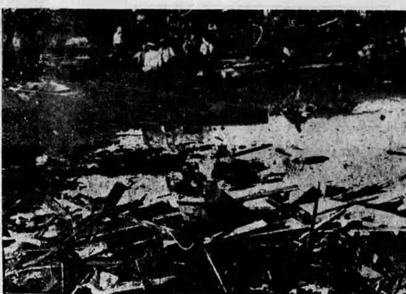
FIREWORKS BLAST KILLS ONE— Fire inspectors, background, examine scene of fireworks warehouse explosion in Portland, Oregon, which razed several homes and shattered windows as far as 22 blocks away. At least one person, a little girl, was killed and more than 20 injured.
