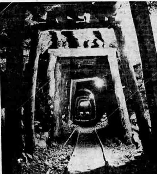
THE SHAFT ITSELF at the Rainbow Ridge mine is about a thousand feet in length at the present time. Tours of the shaft are usually available from owner Keith Hodson. The shoring is native timber.
