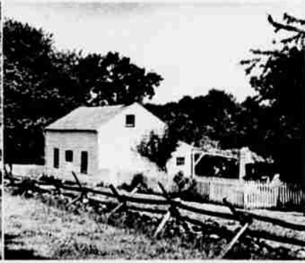
Leister House, which served as General Meade's Union headquarters, still shows bullet holes.
