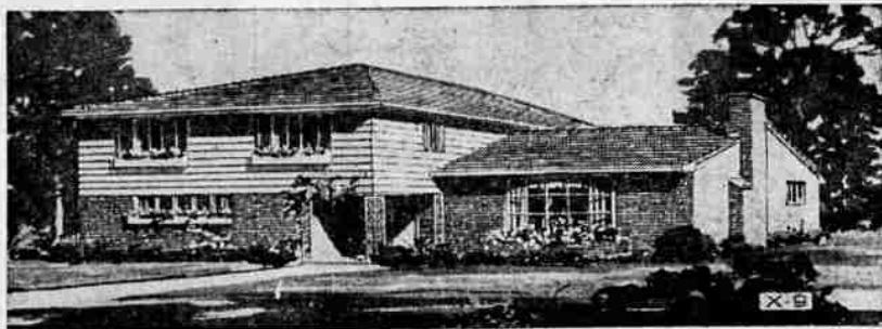
WROUGHT IRON TRELLIS COLUMNS and wood and stone flower boxes greet the visitor to this multi-level "green thumb" house. The arrangement of its levels is based on a technique used by Oriental experts in planning terraced gardens.
