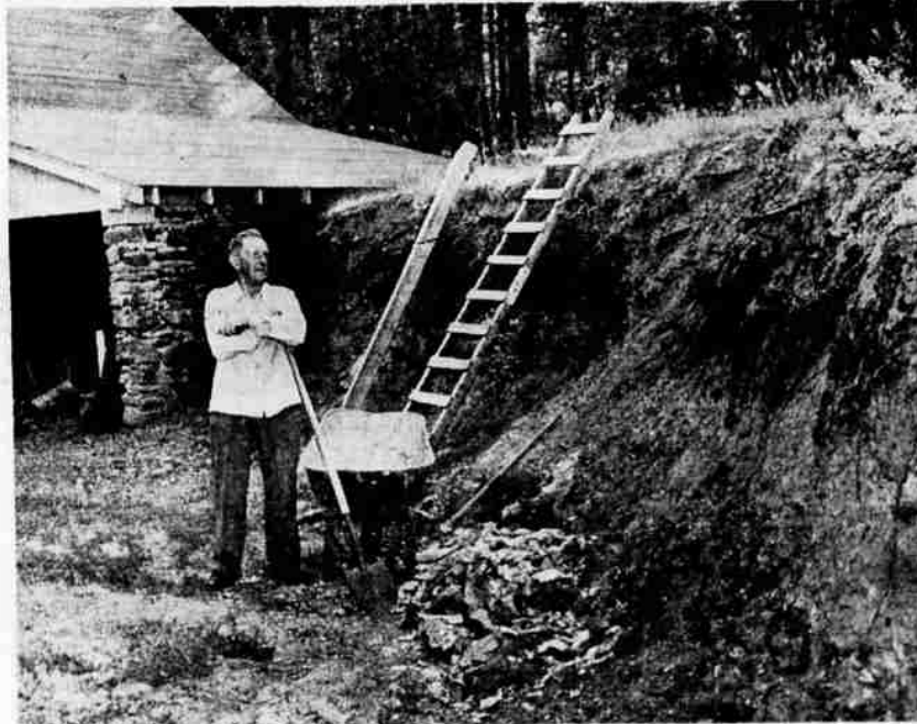
LAND WAS CLEARED of trees and leveled by hand for buildings at Trail's End. Left rear is the garage and woodshed with rock and cement walls built by the couple. A charming small guest house, cozily furnished, is above the garage, reached by wide cement steps. Chokecherry bushes in full bloom along the walkway promise jars of tart jell on pantry shelves next winter. Worn out wheelbarrows and a flock of shovels, dulled by use, are proof that no power machinery lurks in the bushes. Every bit of work has been done by the Von Berthelsdorfs using only hand tools.
