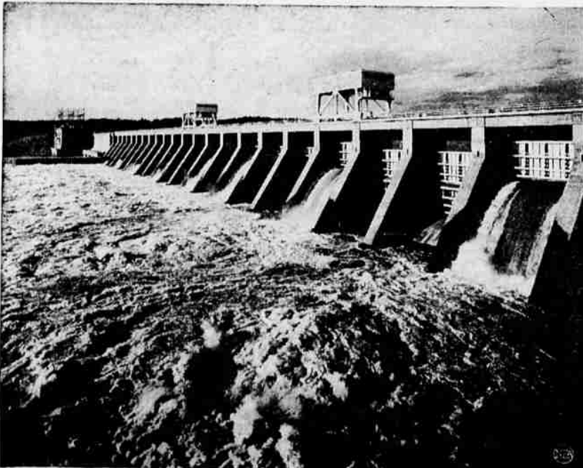
PICKWICK LANDING dam is 113 feet high, 7,715 feet long. Built in 1935-38, its powerhouse has an installed capacity of 216,000 kw. It is one of 31 major dams in TVA, regulating Tennessee River and its tributaries for flood control, navigation development and power production.
