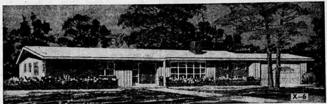
TWO BRICK VENEER PANELS add interest to the exterior and lend solidity to the house. The left panel, fronting the bedroom wing, extends and thickens beyond the end of the house.
