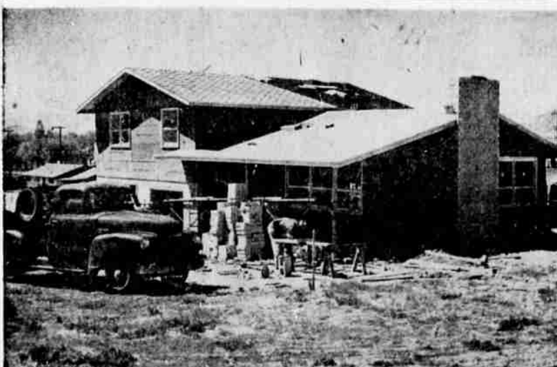
NEW HOME CONSTRUCTION continues high in Klamath Falls and vicinity. Shown here is a new home being built by George Anderson in Madison Heights, at the end of Shasta Way. Building permits in Klamath Falls for 1958 thus far show a slight decrease from last year's figures, but still run well above the average of the 1950-1955 period.
