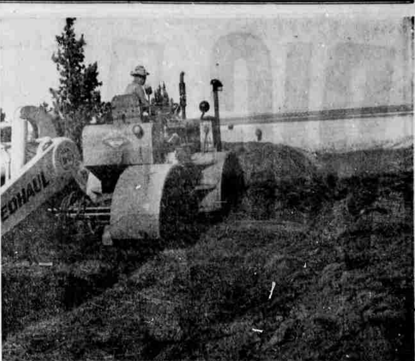
BELIEVING IN FEEDING rather than selling forage crops, the Leonard Pitcher ranch constructed a pit silo last year, the first within the Fort Rock-Silver Lake Soil Conservation District. Jerry Pitcher is shown pressing down forage with a heavy tractor and six yard scraper. —Photo by Parks
