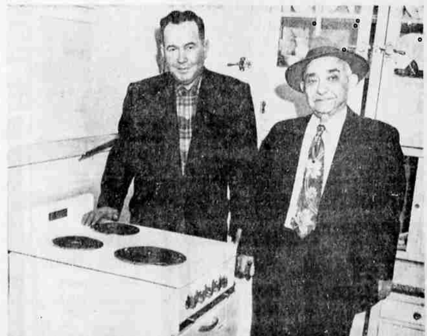
Bob Walker, of Walker Bros. in Merrill, and Christ Blanas, owner of Cascade Apartment Hotel, look over one of the 37 new Hotpoint ranges recently installed in the Hotel.
