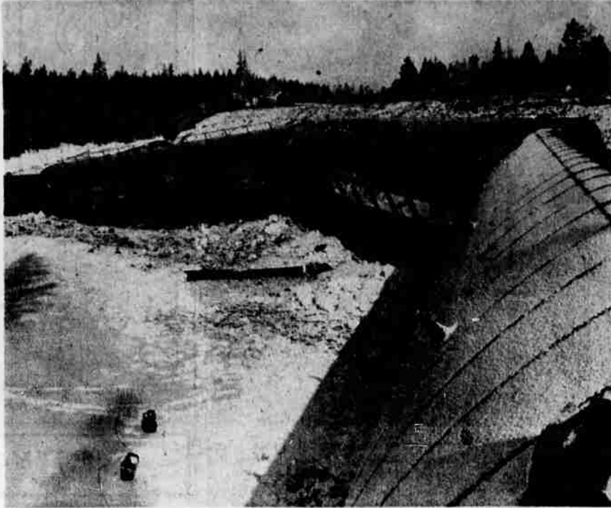
ALTHOUGH 12 out of 14 cars on the Cascade Limited jumped the track early Saturday morning, a miracle seemed to prevail and only one of the cars completely overturned or upended. The overturned car can be seen lying on its side in the far left portion of this picture. The car was occupied by portions of the train crew and none were seriously injured.
