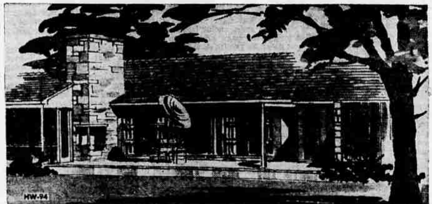
THIS REAR VIEW shows, from left to right, the screened-in dining porch, the barbecue grill and the 30 by 10 foot terrace.
