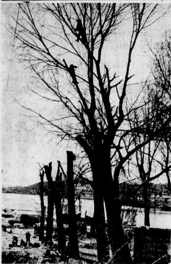
TREE TOPPING in Veterans Memorial Park was performed recently by Copco, who topped seven dead trees adjacent to power lines at the request of the park and recreation department. Department director Bob Bonney said that only alternate trees were topped so as not to destroy all the shade trees. The topped trees will be replaced allowing the new trees to develop as the old ones rot.
