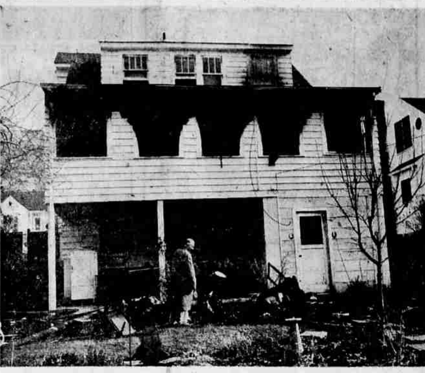
FLAMES ORIGINATING from an undetermined cause near midnight Saturday, caused the death of Dr. and Mrs. Ray W. Oldenburg at their home, 1228 Pacific Terrace. It is believed the couple retired about 11 p.m. and flames were discovered about 30 minutes later in the second story sunporch by passersby. The Klamath Falls Fire Department received the call at 11:29. The body of Mrs. Oldenburg was discovered in a second story bedroom. Dr. Oldenburg had gone to a first floor bathroom and opened a window, apparently collapsing before help reached them. Flames were controlled within a few minutes after arrival of the fire department. Neither suffered burns.
