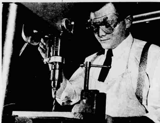
The do-it-yourselfer can protect himself by wearing eye shield and clamping down stock work to bench.
