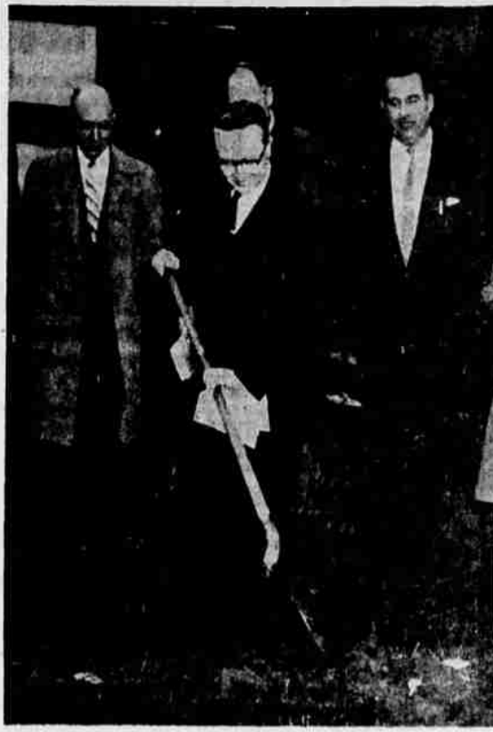
GROUND BREAKING CEREMONIES for the new Methodist Church at Dunsuir were held last Sunday. Actual construction of the first unit of an entirely new church will begin in the spring. The sanctuary and administrative unit will cost about $45,000 and the building committee has been authorized to invite bids. The Rev. O. A. Terrill is shown with the shovel at Lee Huddle, Carl Nelson and Glen Minuth, shown from left to right, look on.
