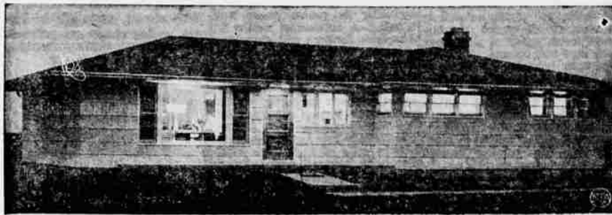
LIGHTS BLAZE a cherry welcome from the windows of this model farm home in the heart of the Illinois farmland. The prefabricated three-bedroom house was a featured attraction at the Farm Progress Show.
