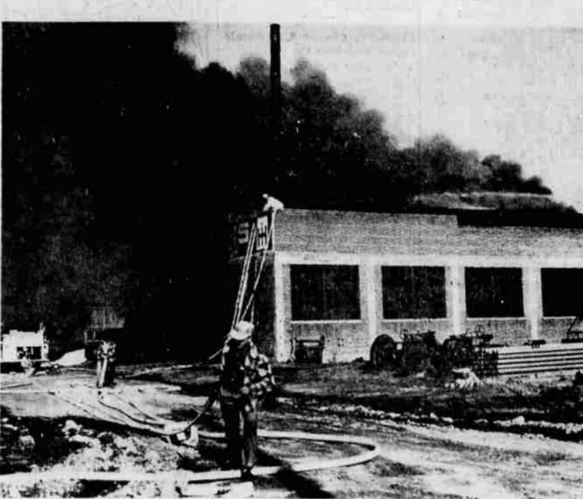
THE J. W. KERNS tractor maintenance shop on South Sixth Street was extensively damaged by fire early Wednesday afternoon after a blaze broke out in the rear portion of the building when gas fumes from a tractor carburetor made contact with an open flame. The fire quickly spread through the false ceiling and into the mezzanine floor where large stocks of tires were stored. City, suburban, and OTI fire crews required one hour and a half to bring the fire under control. In addition to materials, the roof of the building was also damaged.
