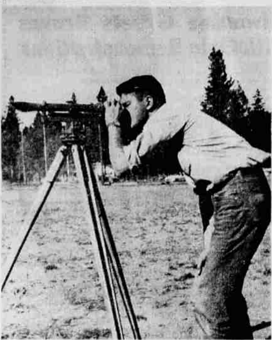
REMO MINATO, Klamath Agency, president of the Reservation Jaycees, is one of three engineers from the agency working to stake and engineer the Chiloquin baseball field for leveling.
