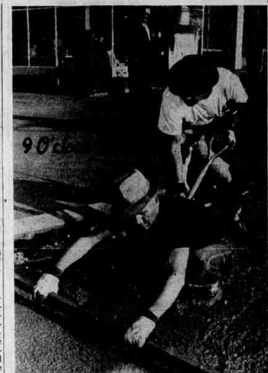
BOB HOLLOWAY, left, and Bill Blind, were almost knee-deep in cement this morning when the 9 o'clock photographer stopped by. The two men, employees of H. O. Sample, were doing work at a Richfield station at First and Main streets.
